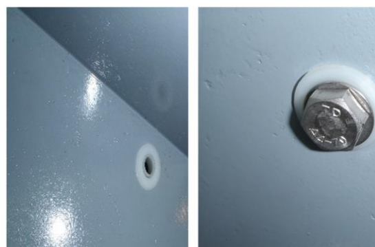
Figure 37 Plastic insulation between different metals
