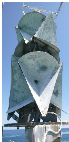
Figure 41 Damaged coating
